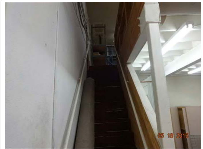
15. View of stairway leading to second level.
