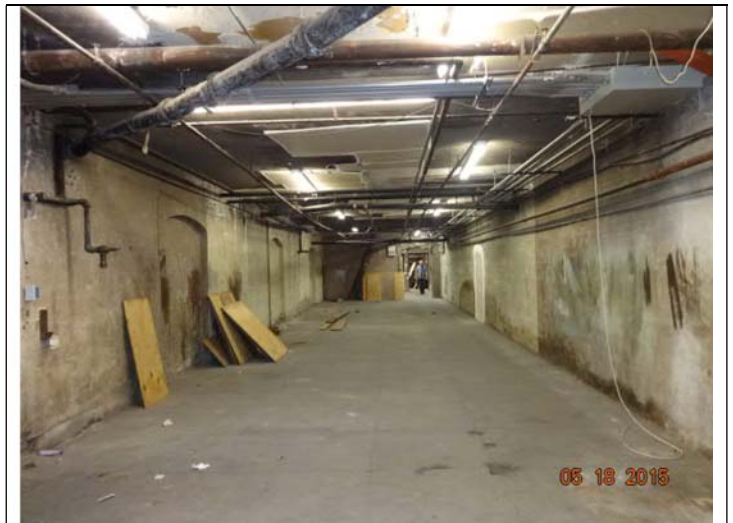
22. View of basement level warehouse area.
