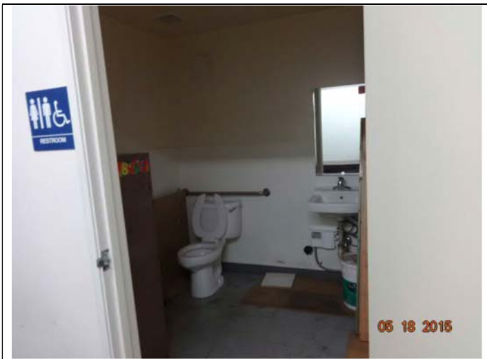
17. View of typical employee restroom located at the subject property.
