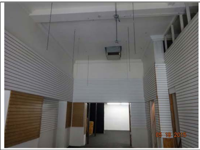
19. View of typical vacant unit.
