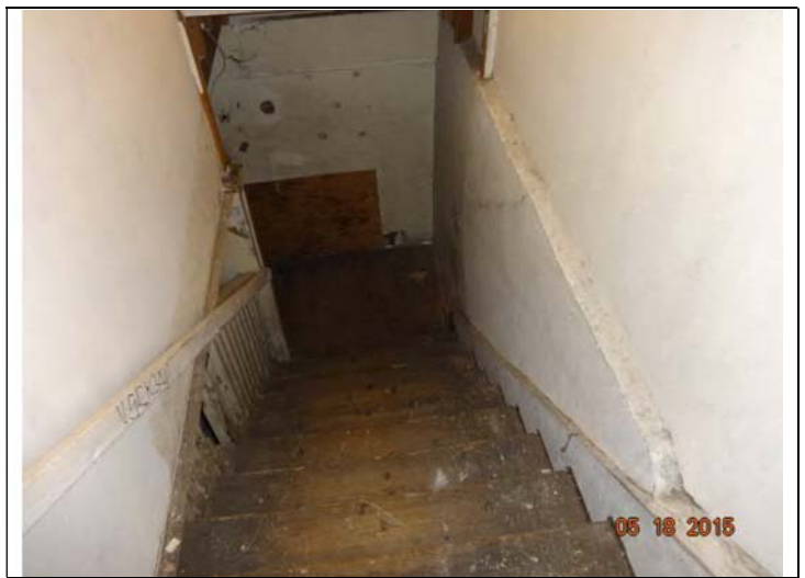
20. View of stairwell leading to a basement level.
