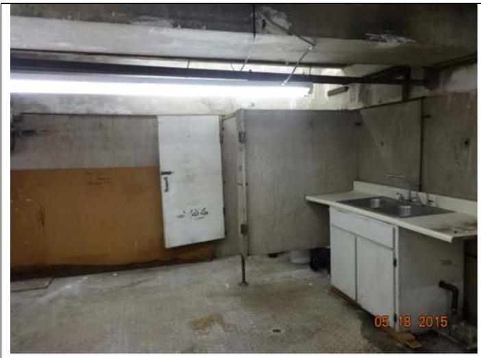
21. View of basement level restroom.
